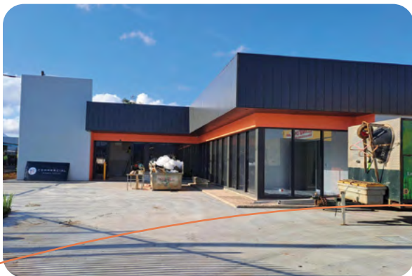
Above: Royal Rehab LifeWorks Cairns hub under construction.
